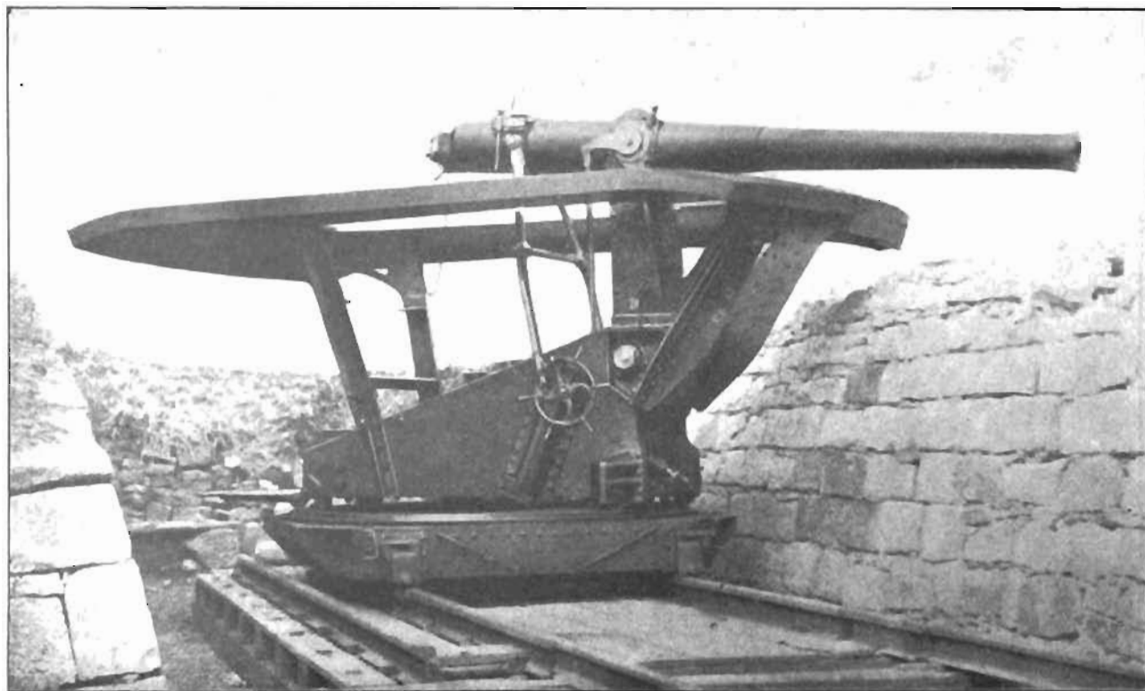
120 MM. GUN (DISAPPEARING CARRIAGE), ON RAILWAY MOUNT USED BY THE SWISS GOVERNMENT FOR THE DEFENSE OF THE RHONE VALLEY.
