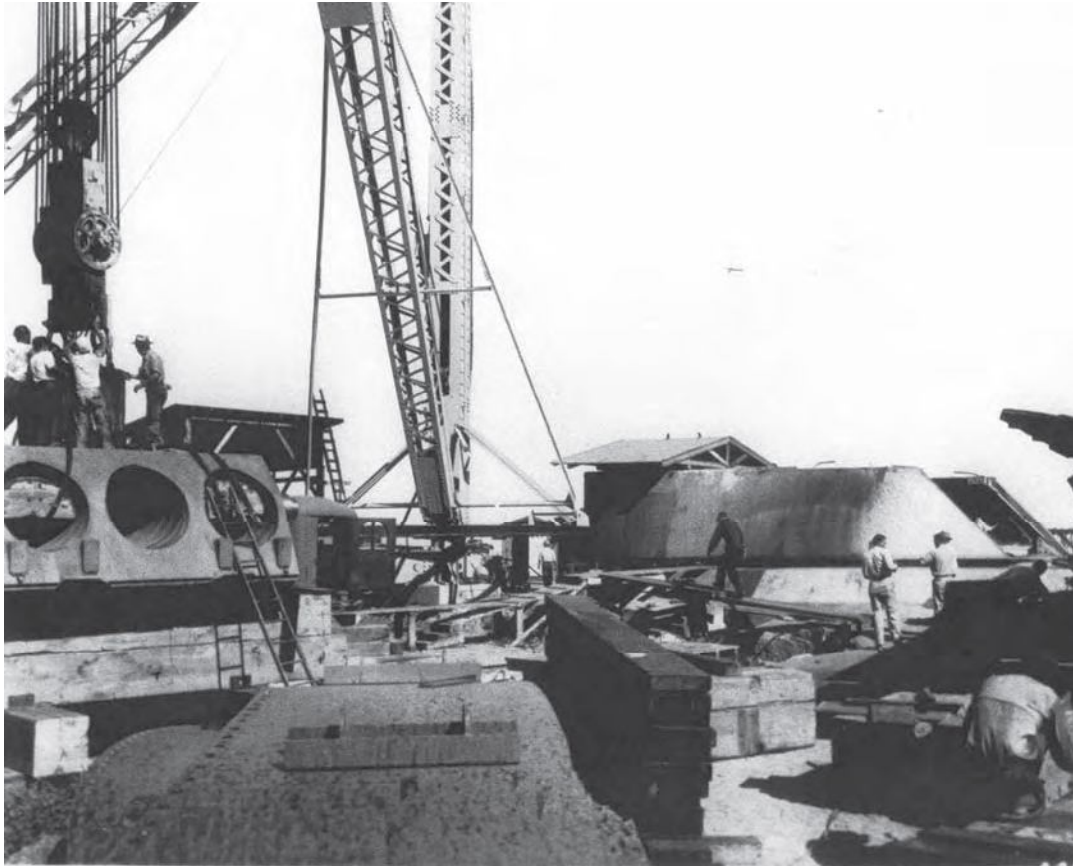
Assembly of turret at Battery Pennsylvania showing heavy-lift derrick. USAMH
