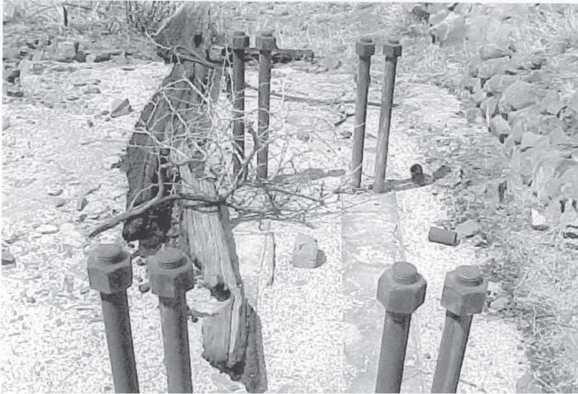
Concrete footing and heavy-duty mounting bolts. Author, 2000.
