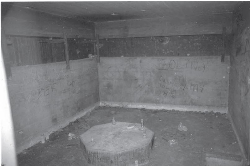
Interior of the BCS showing concrete pier for DPF pedestal. Bolling Smith
