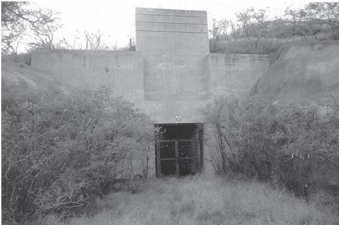
No. 2 Portal showing ventilator stack and gunite applied to both sides. Bolling Smith, 2000
