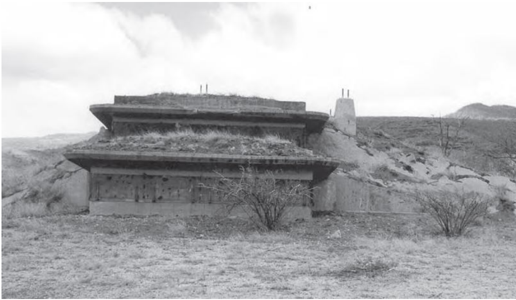
Battery Arizona's BCS showing closed shutters and mounting piers for SCR-296A radar. Author, 2000
