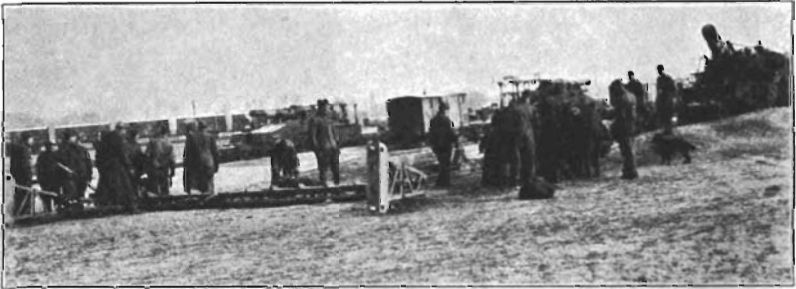
BRIDGE SPAN READY FOR ERECTION.
