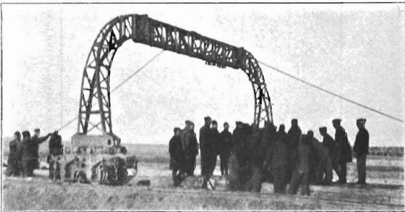
SETTING UP ROLLING BRIDGE.
